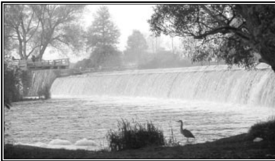
Edmonds Dam - Rideau Canal Photo Collection
