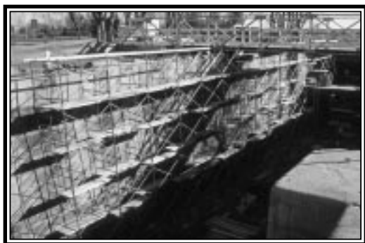
Scaffolding in the upper lock at Long Island, Bill Pratt
