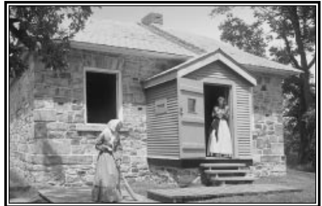
Sweeney House at Jones Falls - Rideau Canal Photo Collection
