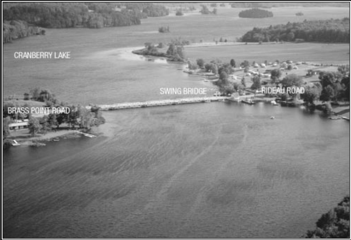
BRASS POINT BRIDGE
