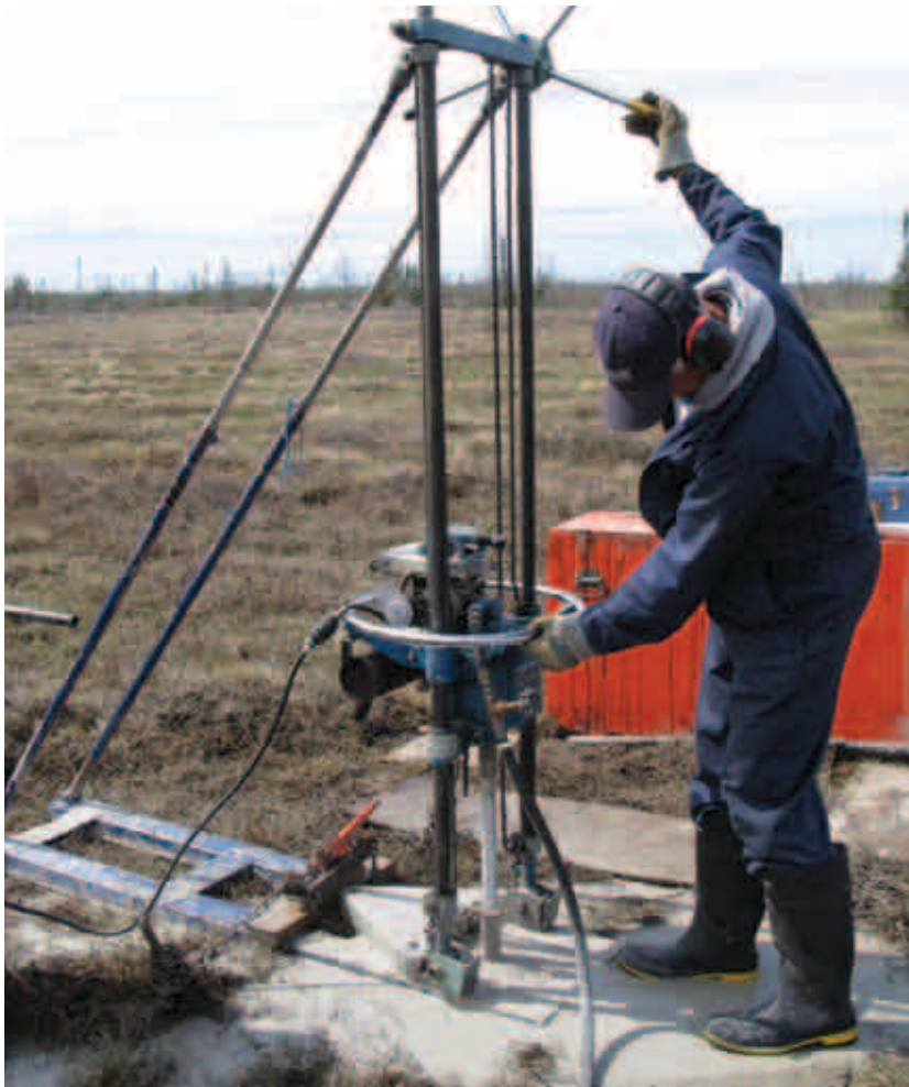
Lightweight diamond drill used for installing thermistor cables. Credit: Wendy Sladen.
