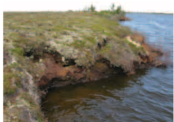
Thawed and collapsing peat bank by Fletcher Lake. Credit: Larry Dyke.
